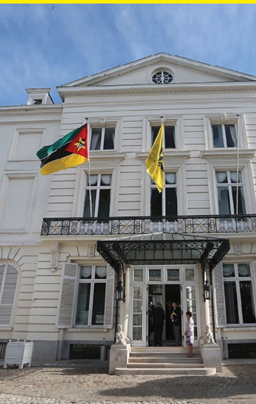
The Errera House in Brussels, the official residence of the Government of Flanders.
